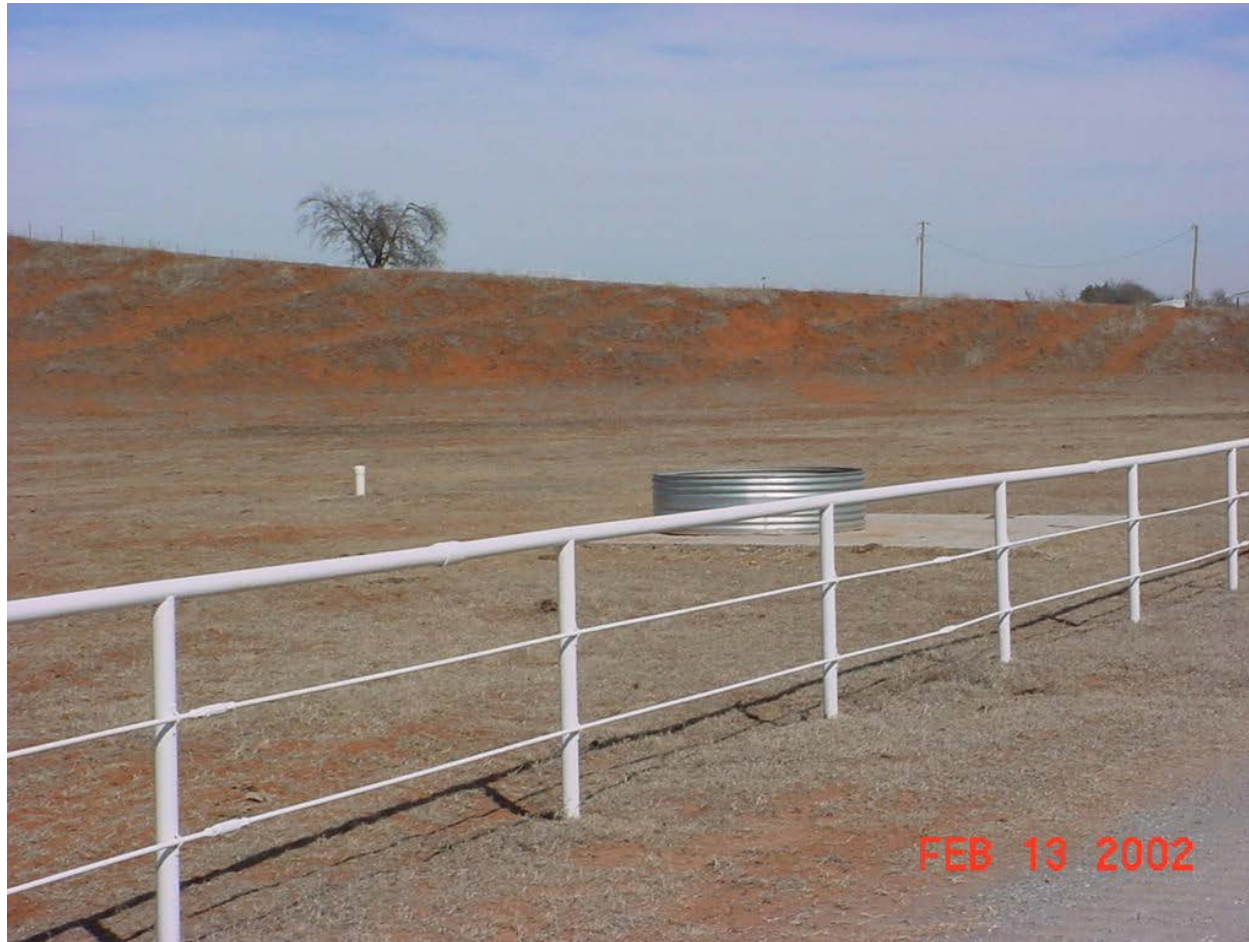
Structures in Auxiliary Spillway
