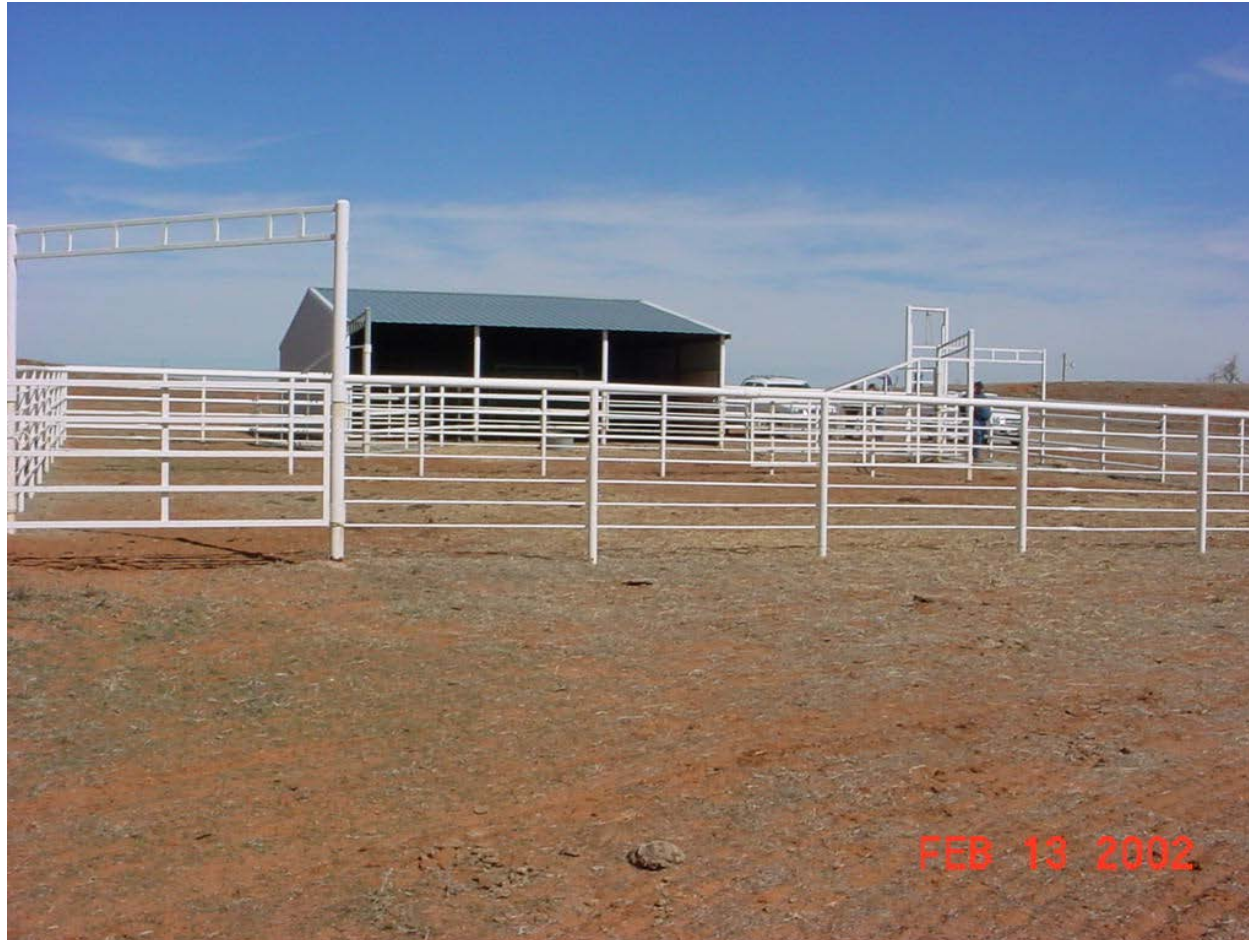
Structures in Auxiliary Spillway
