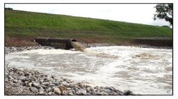
Water is released through a pipe in the dam for several days after a heavy rainstorm.
