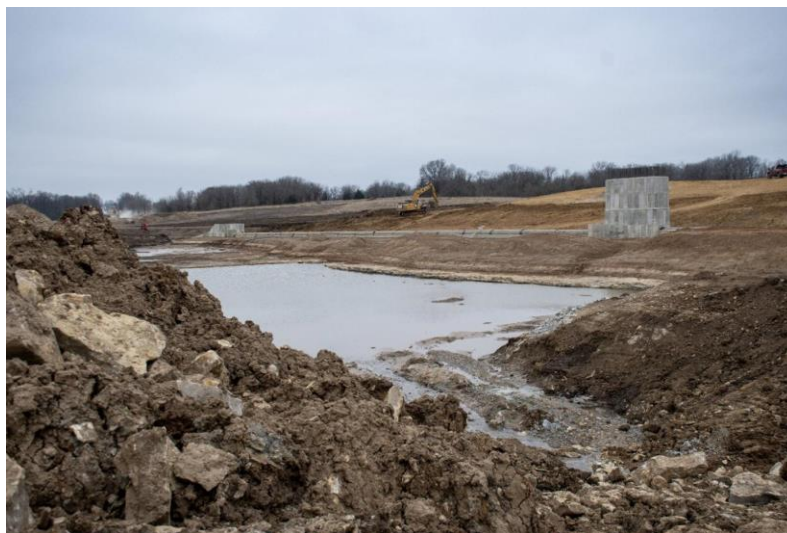
Construction of Little Otter Creek Dam – photo credit Joshua Colligan, NRCS-MO
