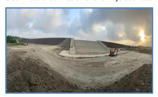
A roller compacted concrete spillway was constructed as part of the rehabilitation project.
