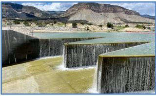
The auxiliary spillway at the Millsite Dam shown here on June 20, 2023, was originally constructed in 1971. The recently completed rehabilitation project of the dam included a complete reconfiguration of the auxiliary spillway.
