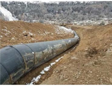
Fire Mountain Canal Improvement Project – New siphon entrance and screen structure (left) with HDPE piping related to segment 47 pipeline (right) is one example of the seven off-farm projects funding through the RCPP.
