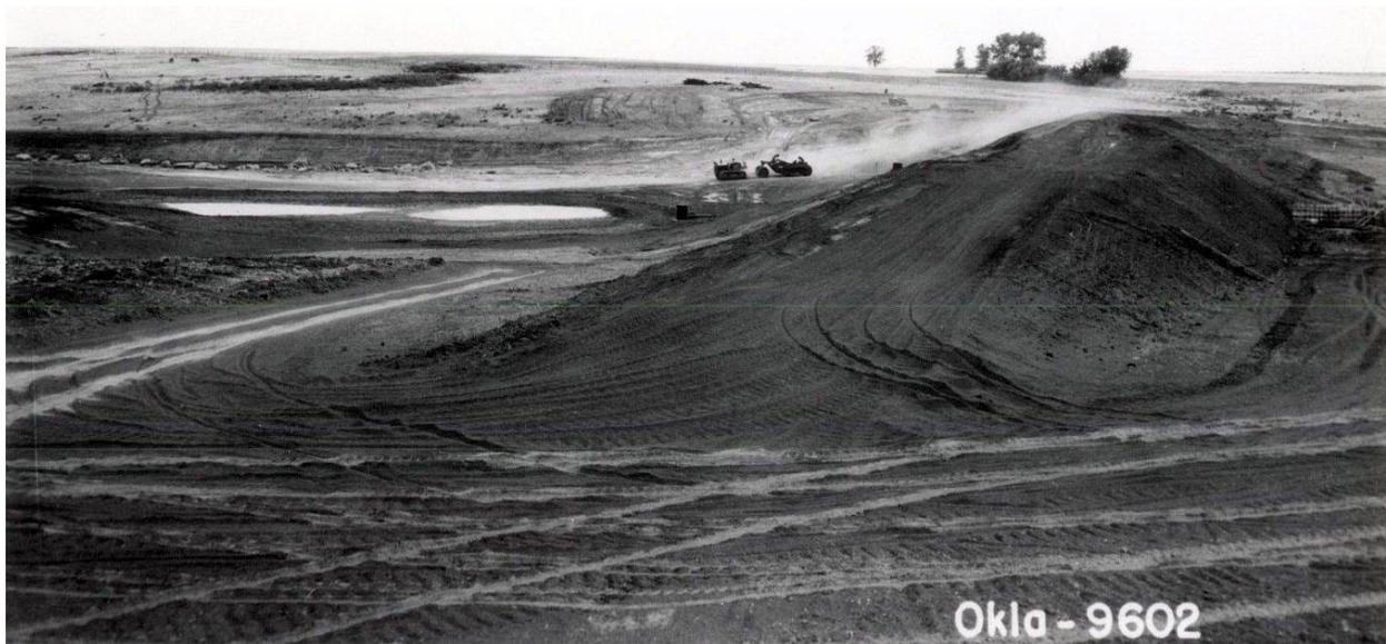
Photograph from May 1948 showing construction of the detention dam for Cloud Creek Reservoir No. 2, which was completed about the same time as Cloud Creek No 2. Together these two reservoirs on Cloud Creek would serve to contain excess runoff from heavy rains, catch sediment from flowing downstream, and provide numerous benefits to surrounding communities. ([Oklahoma Conservation Historical Society Photography Collection](#))
