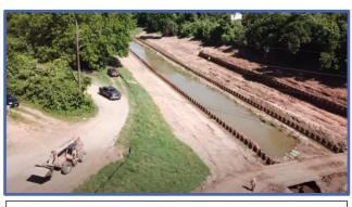
Steel sheet piling 20 to 30 ft deep was installed to stabilize the ground and riprap concrete blocks installed to prevent future erosion.
