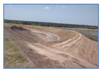
A coffer dam was constructed during the rehabilitation of the dam to allow the construction of a roller compacted concrete spillway over the earthen dam.
