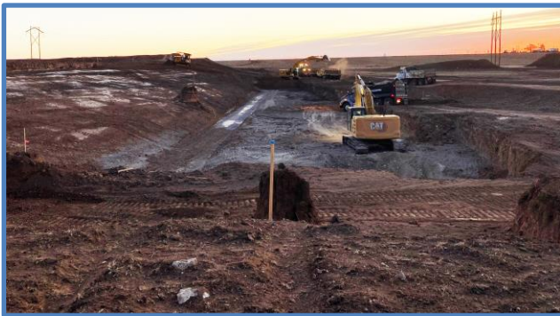
Dam under rehabilitation in June 2023
