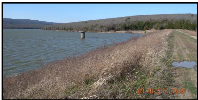
Dam prior to rehabilitation
