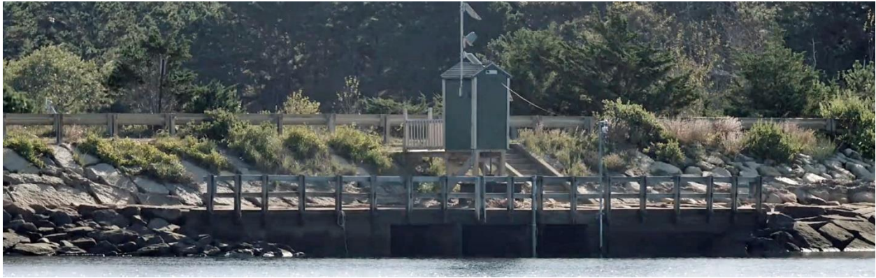
Existing dike constructed in the early 1900's
