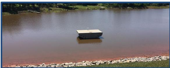
A new concrete inlet tower and concrete conduit was installed during the rehabilitation project.
