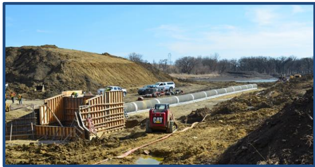
A new principal spillway was constructed through the dam.
