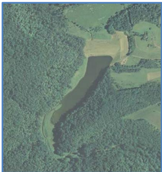
Dam before rehabilitation
