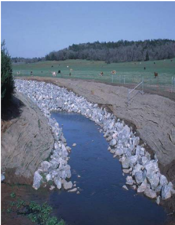
Figure 6. Grade Stabilization, Gracemont, Oklahoma
