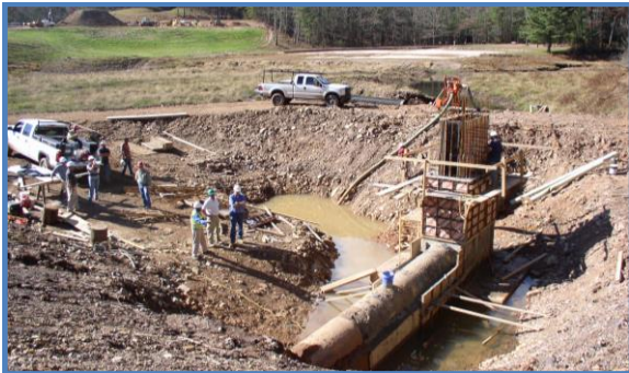
The concrete principal spillway inlet tower and gates were replaced.
