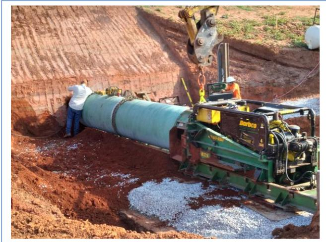
A new concrete pipe was installed using a “jack and bore” technique.
