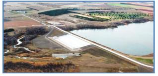
The project included raising the height of the dam and installing a roller compacted concrete spillway in the center of the dam.
