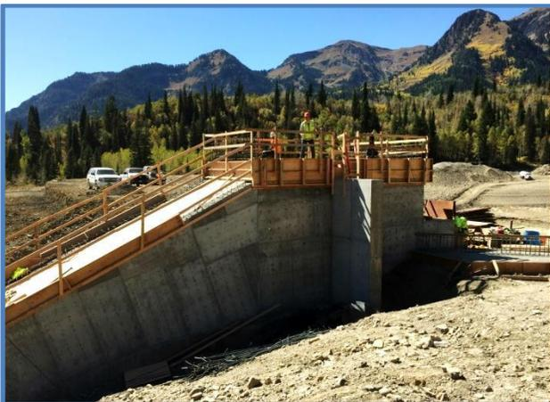
A new auxiliary spillway was constructed during rehabilitation of the dam.
