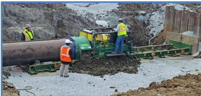
The principal spillway pipe was replaced on Rock Creek Dam No. 16 during rehabilitation.
