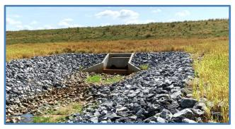
A new outlet channel and impact basin was constructed as part of the rehabilitation project.
