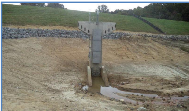
The principal spillway riser was replaced during the rehabilitation project.
