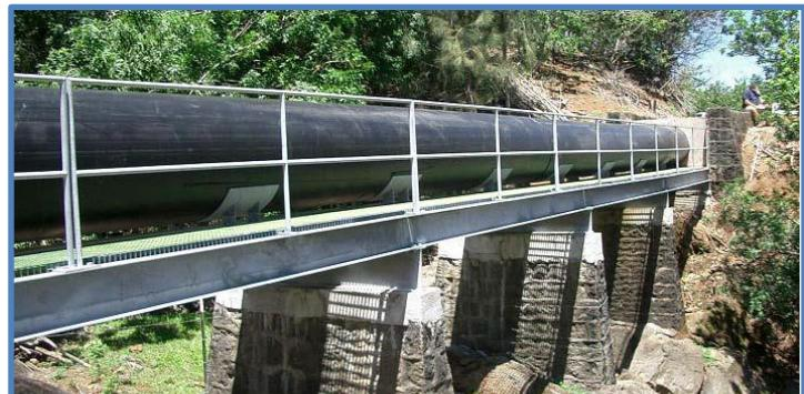
Local sponsors developed the Lower Hamakua Ditch Watershed Project on the island of Hawaii to rebuild and repair a water distribution system that had been built by sugar companies in 1900-1910. The 15 miles of open ditch and 10 miles of tunnel provide irrigation water distribution to 8,000 acres of agricultural lands. This flume replaced an existing one that had deteriorated.
