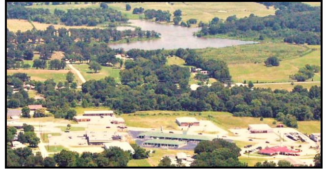
A low hazard dam is reclassified to high hazard when downstream development creates the risk for loss of lives if the dam were to fail.
