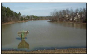
A concrete inlet tower (might be metal on older dams) connected to a pipe extending through the dam serves as a principal spillway for dams, controlling the water level. A slide gate at the bottom of the inlet can be opened to lower the water level for maintenance and repair.
