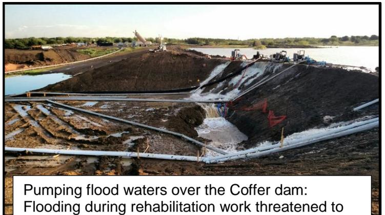
Pumping flood waters over the Cofferd dam: Flooding during rehabilitation work threatened to break the temporary cofferdam.
