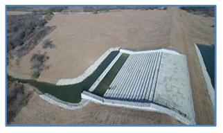
Rehabilitation included construction of a rollercompacted concrete auxiliary spillway.
