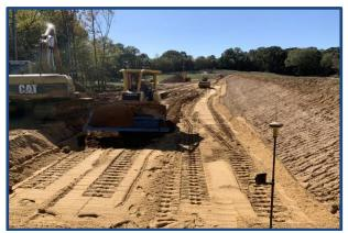
A sand diaphragm will run the length of the dam to protect the dam from a large earthquake event near the New Madrid seismic zone
