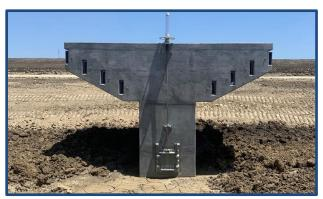
A new principal spillway has been installed during the project.
