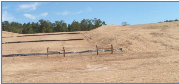
The earthen auxiliary spillway was lowered in elevation and widened.
