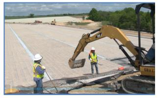
Rehabilitation included widening the auxiliary spillway and armoring it with articulated concrete block armoring.
