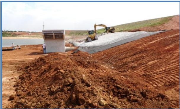
The principal spillway inlet tower and concrete pipe through the dam were replaced during rehabilitation.
