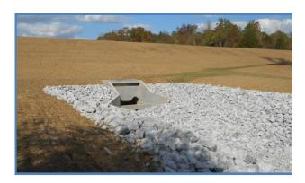
A new outlet channel and impact basin was constructed as part of the rehabilitation project.
