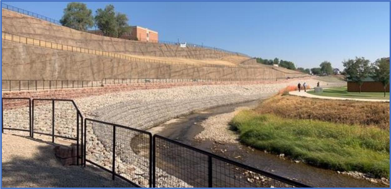
Landslides from a hillside above Goose Creek and the Sheridan Wyoming Junior High School had been a hazard for several years. A retaining wall was constructed about five years ago, but was not successful in fully controlling the hillside movement. High rainfall events had caused the landslide to accelerate and was putting the school and the city at risk from flooding from Goose Creek.
